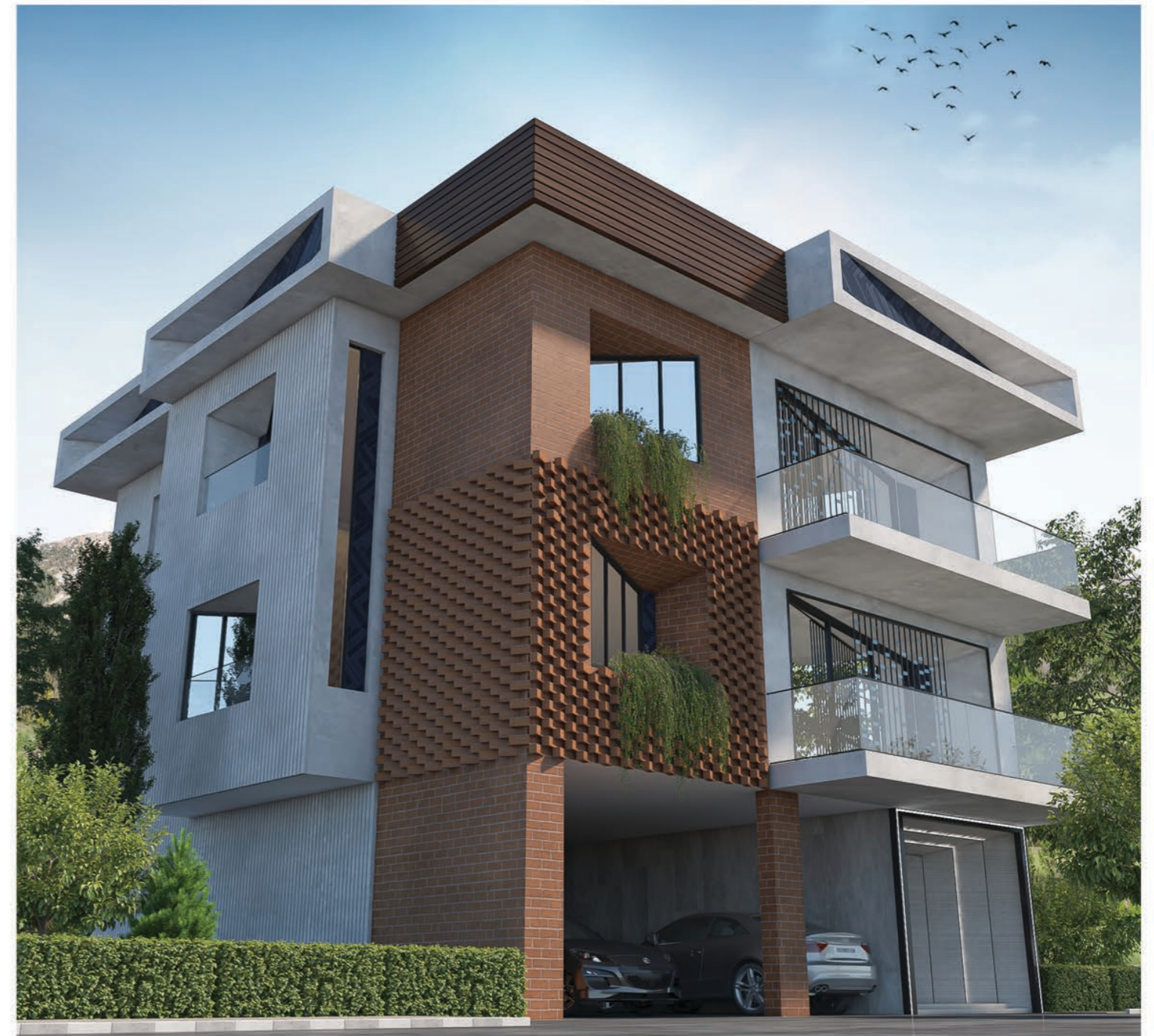
sadaf building architect ali haghshenas location kish island client mr golzari date design 2020
